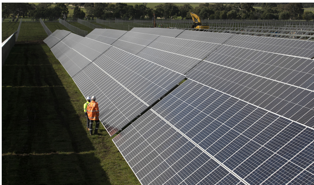
Solar panel installation at Melbourne Airport
