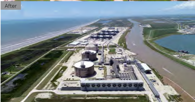
After five years of construction, Freeport LNG is one of the largest and most environmentally sustainable LNG facilities in the world.
