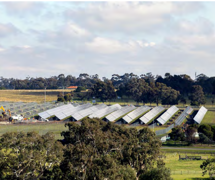
Photo: Solar array development, Melbourne Airport, Australia. Credit: Fiona Hamilton
