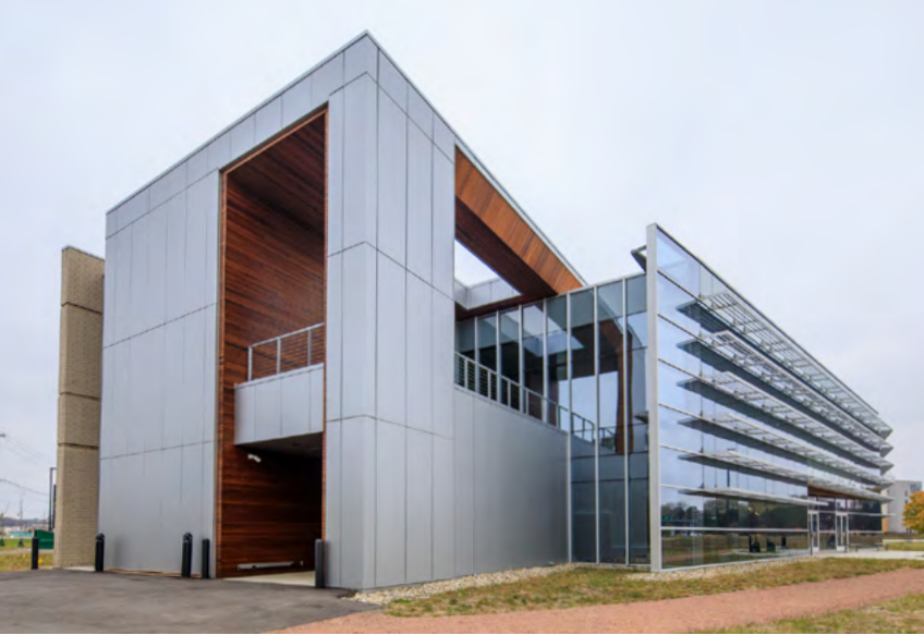
Indiana Toll Road administration building, US
