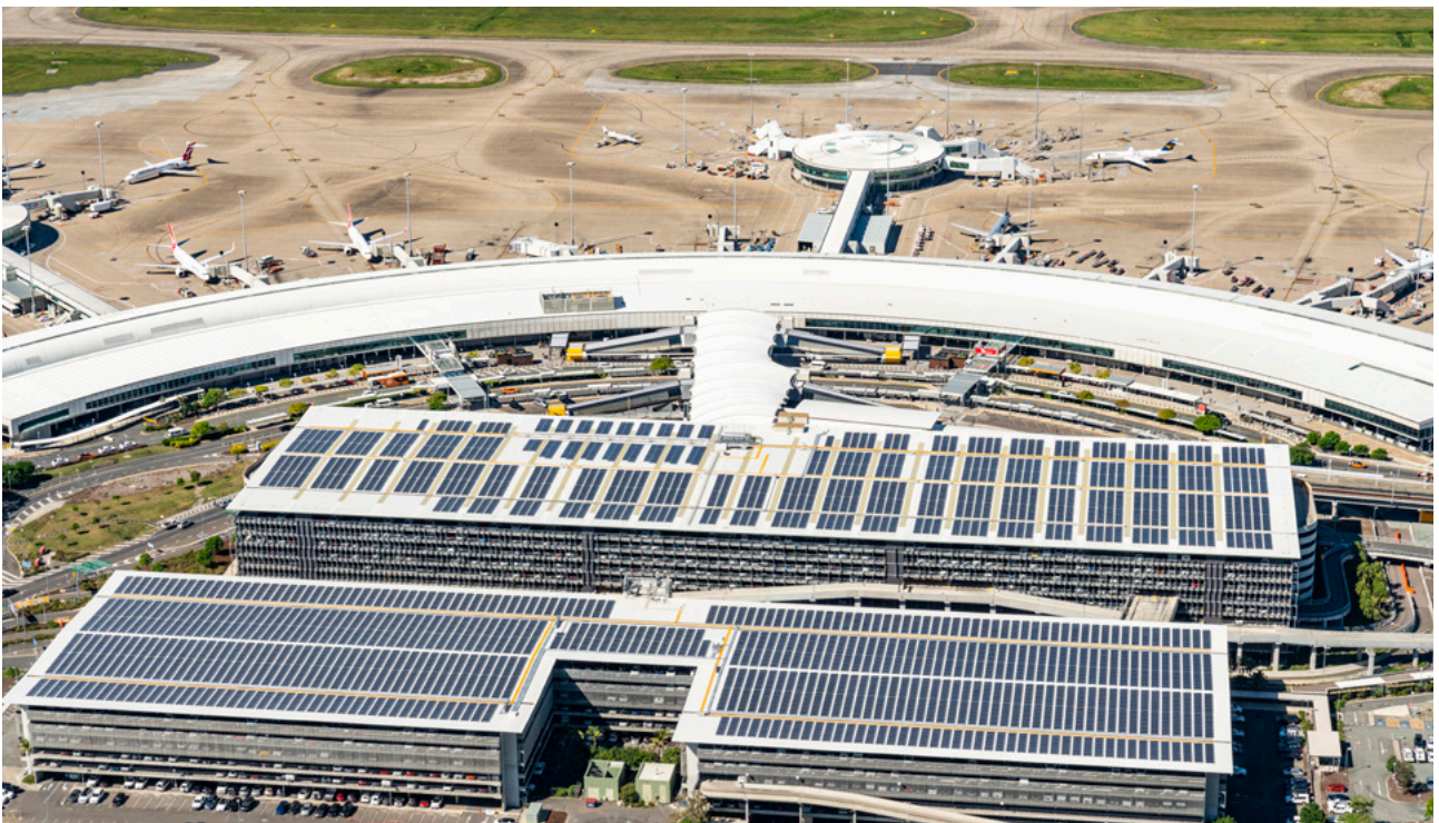
Solar panels at Brisbane Airport
